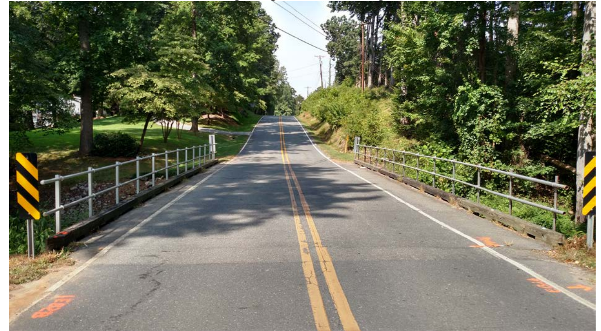
View of Existing Bridge No. 170 Looking Downstation
