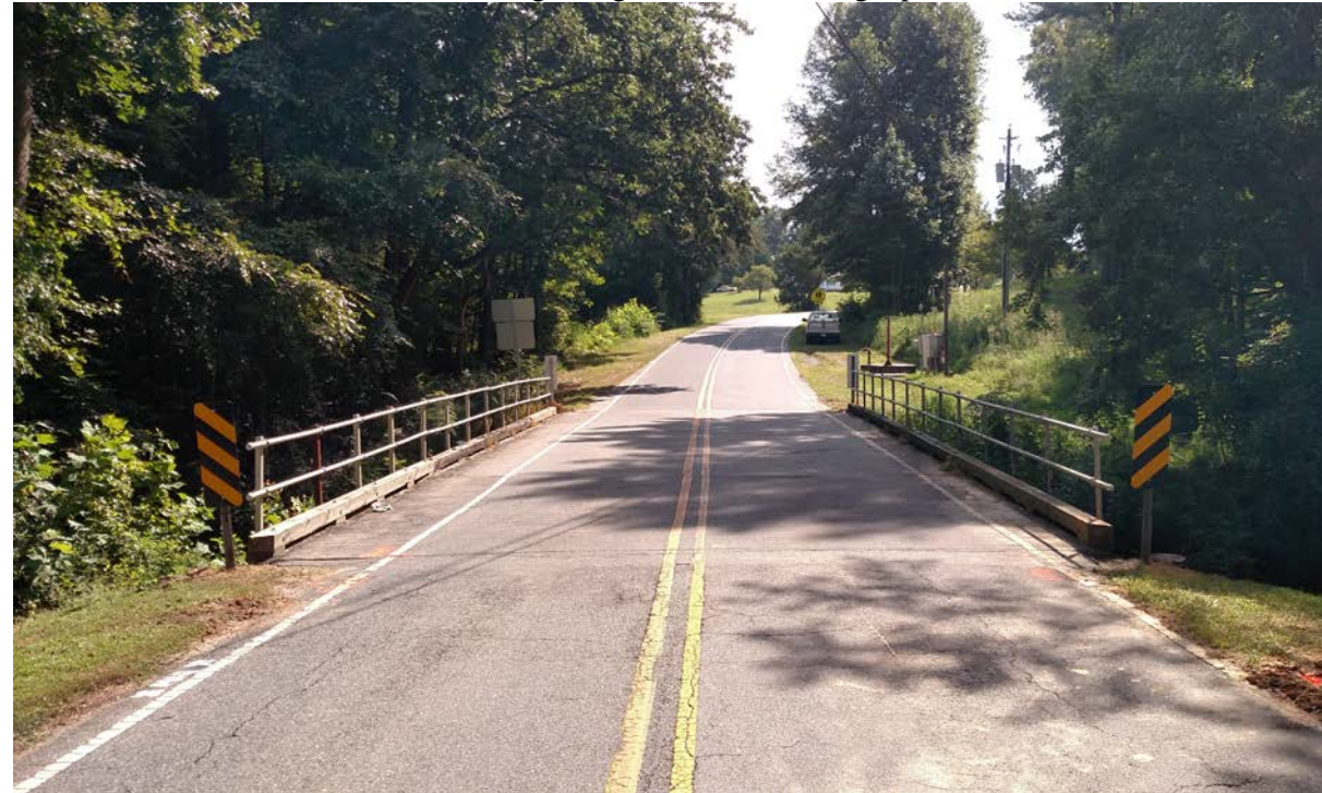
View of Existing Bridge No. 170 Looking Upstation
